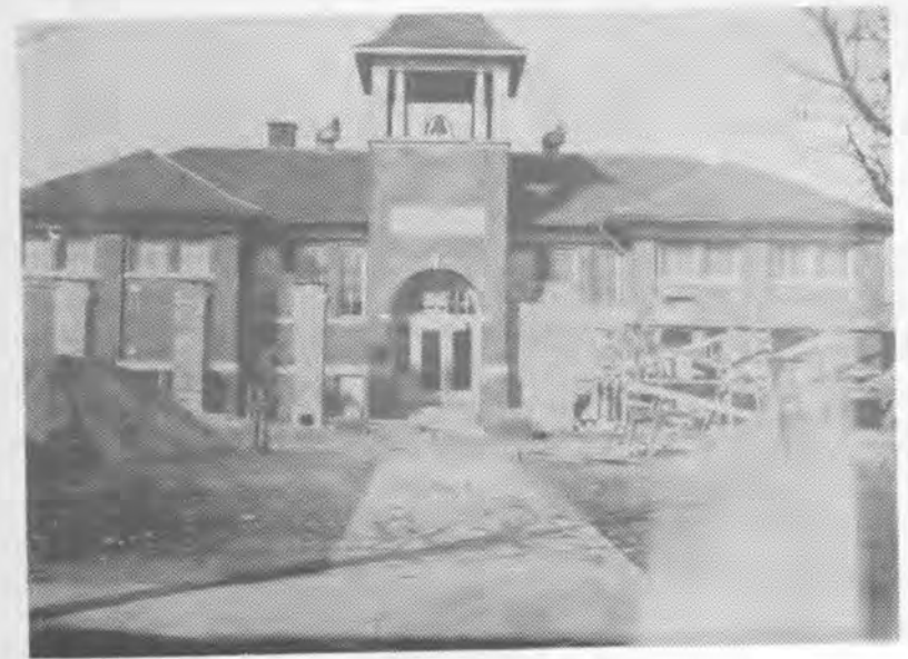
Old High School and Intermediate when being built.
