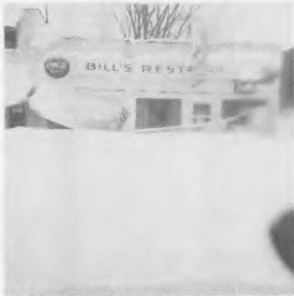
Damage to Bill's Restaurant from big Snow fall - January 1967
