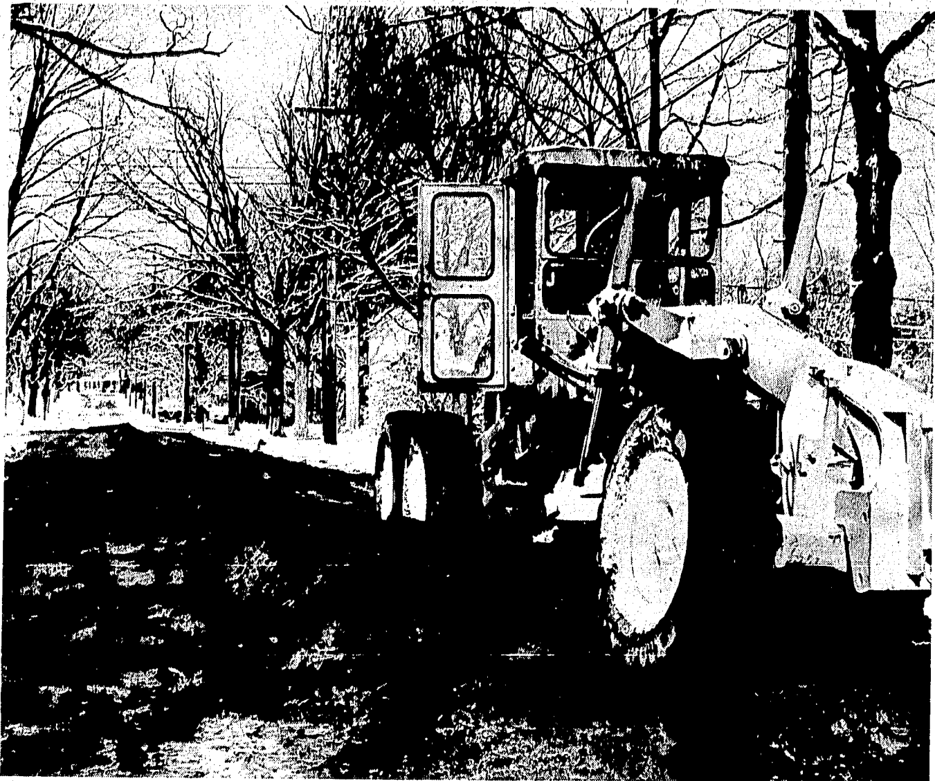
SMOOTHER SAILING --Motorists traveling the one block section of McRoberts street between Ash and Maple streets will find the ride a bit smoother. Workmen were authorized to dig up existing paving and replace it with gravel. Condition of the paving was such that it was impossible to repair the chuck holes and have the patches hold. The job took workmen one afternoon and hopefully there will be funds to get the street re-paved in the near future.
