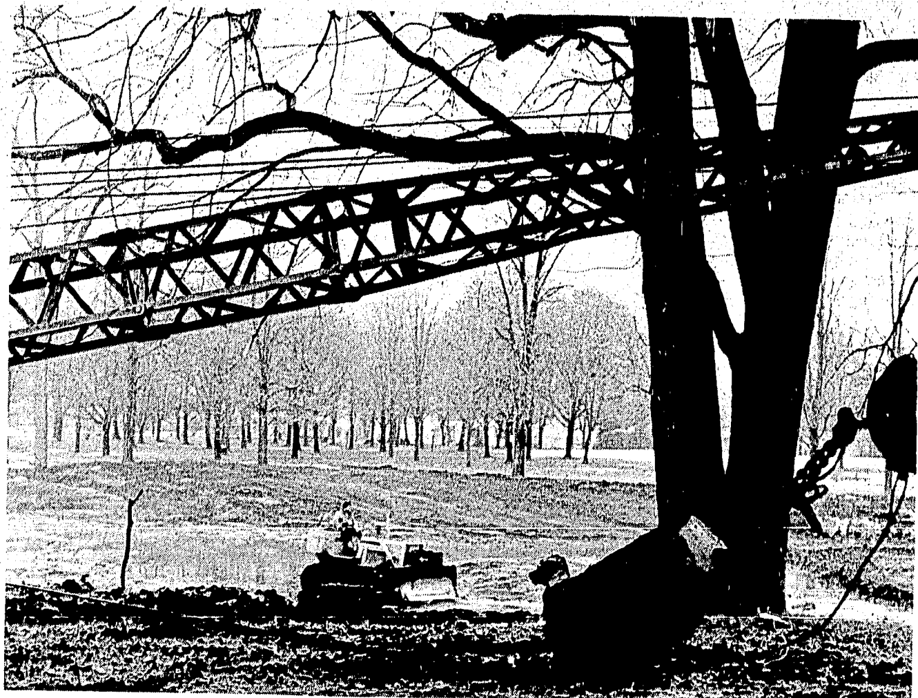
MUCH NEEDED IMPROVEMENT--For years the Rayner Park ponds have been dying a slow, painful death through the cycle of nature and the carelessness of man. Personnel of the Ingham county road commission drained the ponds some time ago and have now begun to scrape the sludge and debris from the bottoms of the ponds. All this is being financed through available funds with the end result to be cleaner, more enjoyable ponds next summer to compliment the park facility.
