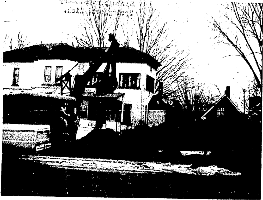
GROUND IS BEING BROKEN here for the new Peoples State Bank building in Williamston. The bank site is in the yard of the James Leasia property. The house in the background was built by Dr. James Leasia in the early days of the village. Dr. "Jim", the town's first doctor came to Williamston in 1840. The location was purchased from the granddaughter Katherine Webb Hull, St. Augustine, Florida.
