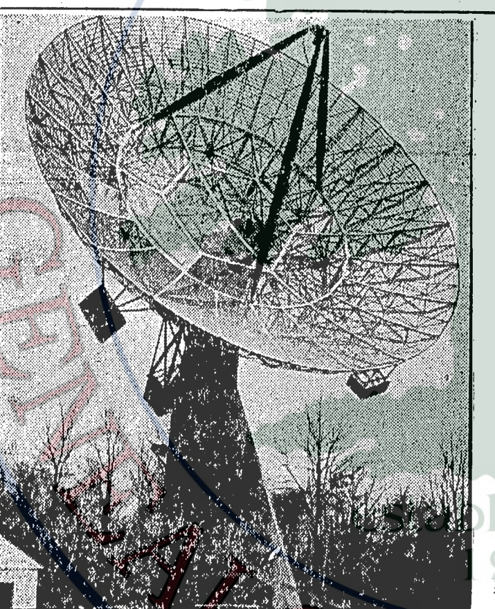
LISTEN TO THE STARS —That's what Harvard's astronomers plan to do with this 60-foot diameter radio-telescope at Agassiz Station, Mass. Largest in the United States, the "ear" is designed to pick up electrical impulses from stars as far as hundred million light years into space. (A light year is equivalent to the distance traveled by a beam of light in one year at the rate of 186,000 miles per second.)
