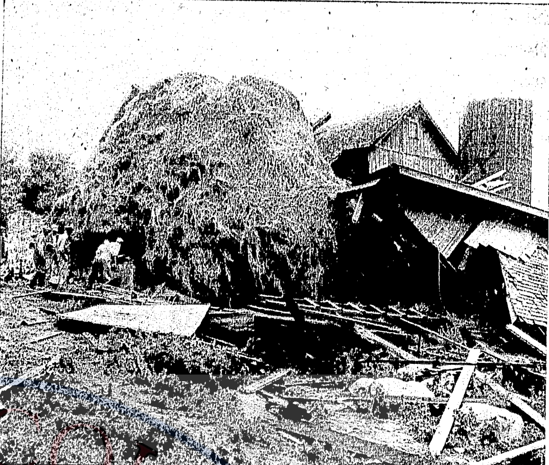
WIND WRECKED THIS BARN on the Jay Coffey farm six miles south of Mason Monday night. Burnett and Burton Coffey and another boy Jim Miller had just left the barn when the building was twisted into wreckage. Helping rescue Coffey's dead hogs are Jay Coffey, Burnett Coffey, Dale Bray, Frank Greener and Dorr Cady. The barn was partly covered by insurance.
