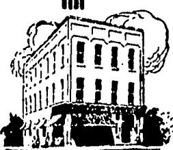
The Bank on the Corner
