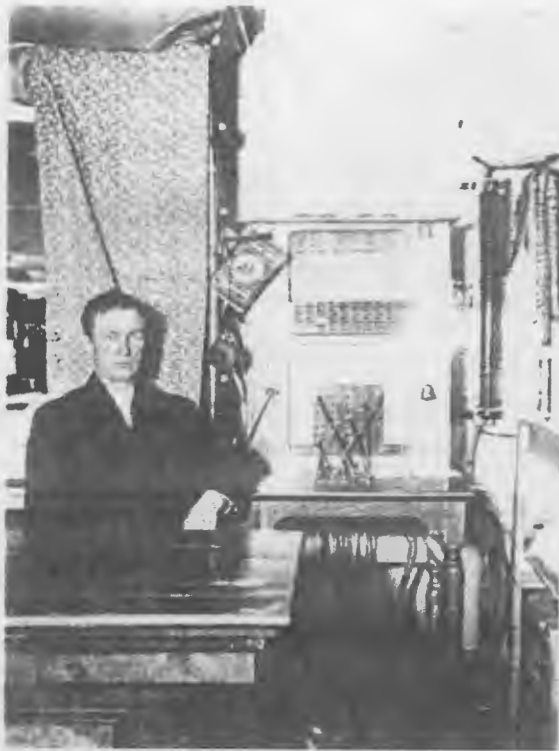
Edward Carley at the switchboard in Munith
