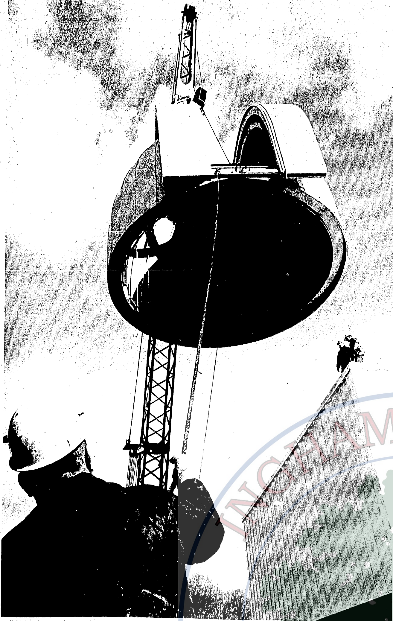
MSU TOP JOB — The rotating dome for Michigan State University's new observatory is lowered into place by workmen. The dome will house a 24-inch aperture reflecting telescope, expected to be installed in a few weeks. The new $660,000 structure, to be operated by the MSU astronomy department, is expected to be operational in three or four months. The observatory is located off Forest and College roads, about a mile from the center part of the East Lansing campus.
